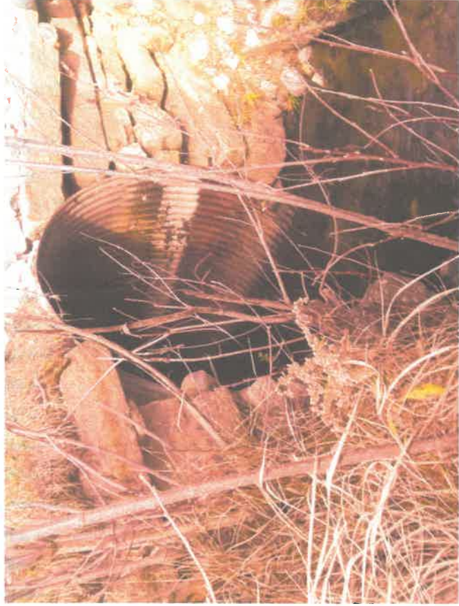
around the Pond Rd. (near Morse Rd./Greenwood Rd.) 72" CMP - POOR
