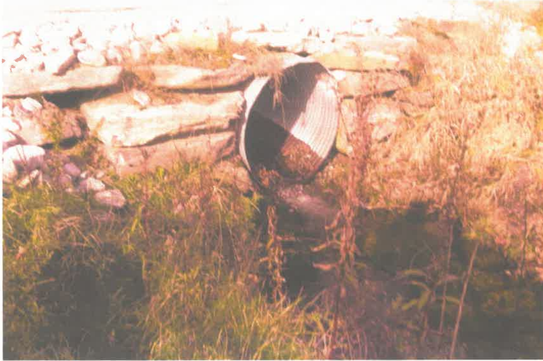
Round the Pond Road Stream Crossing (At Greenwood Road Intersection)
